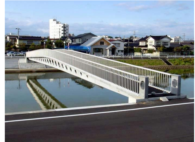
Sakata-Mirai bridge, Sakata, Japan
