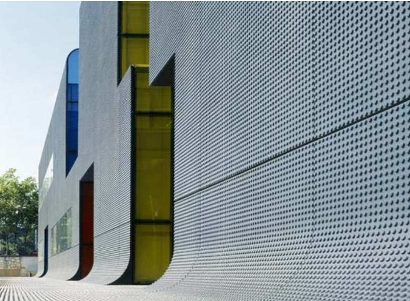
The RATP Bus Depot, Thiais, France
