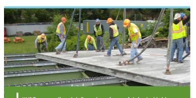
UHPC connection details make using prefabricated bridge elements simpler and more effective for accelerated bridge construction.
