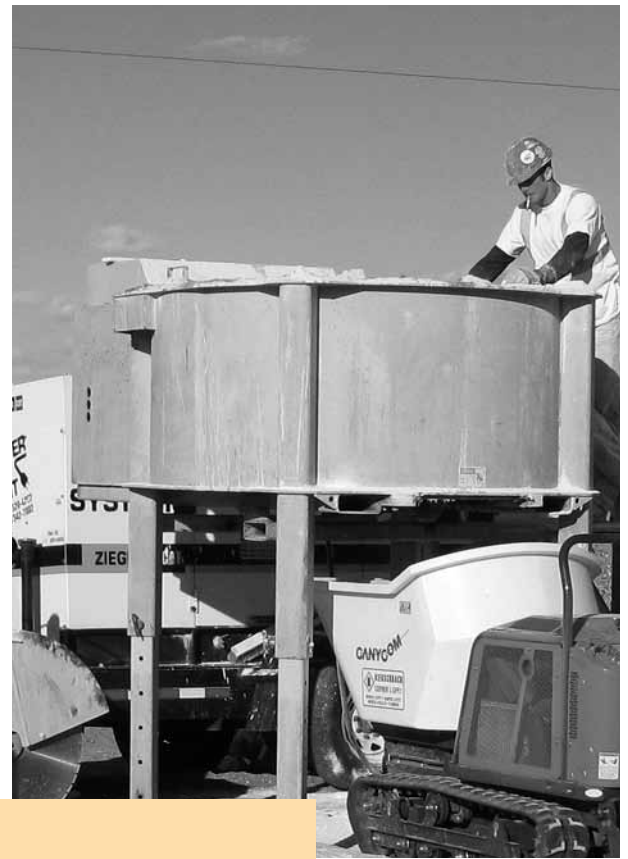
Above: Field-cast ultra-high performance concrete (UHPC) connections were used to construct the Route 31 Bridge in Lyons, NY.
