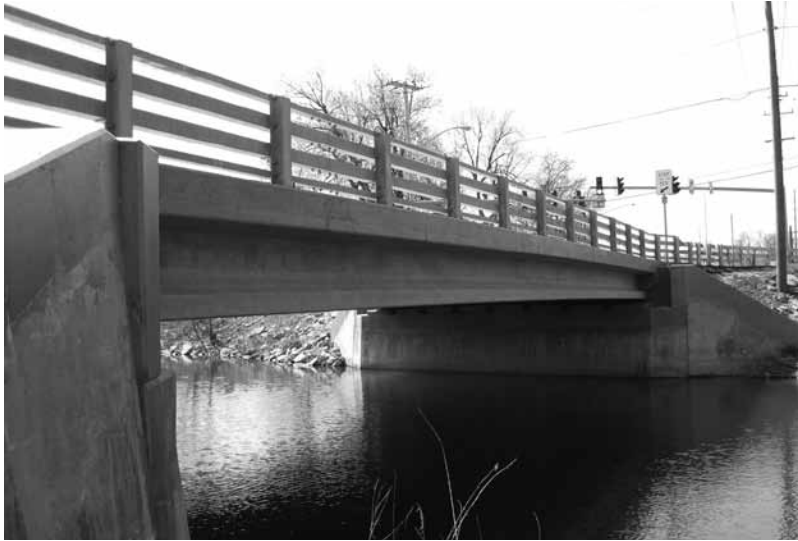
Above: Field-cast ultra-high performance concrete (UHPC) connections were used to construct the Route 31 Bridge in Lyons, NY.
