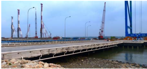
Fig. 1. Bridge25 using UHPC precast beams.
