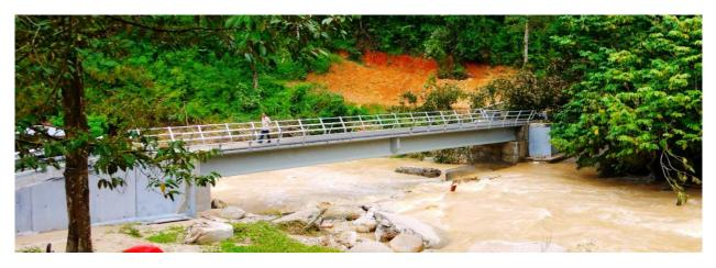
Figure 1 – A 25m single span medium traffic bridge crossing Sungai Itek (Kg. Ulu geroh, Gopeng, Perak) using two pieces of DURA® TBG1325.
