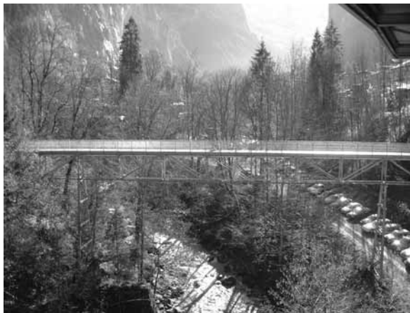
Figure 5: General view of Lauterbrunnen footbridge
