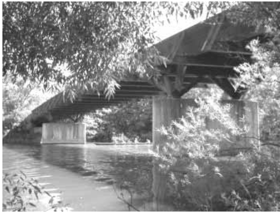
Figure 3: Existing wooden bridge
