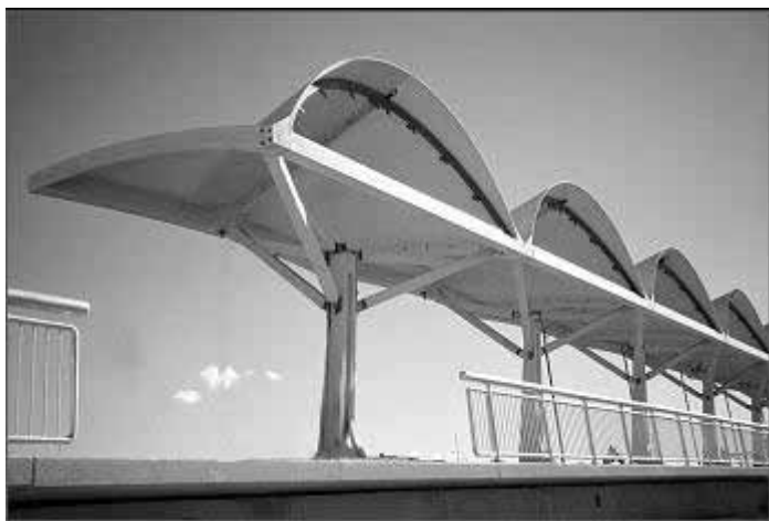
Figure 10. Ductal®-FO canopies - LRT Train Station, Shawnessy, Canada, 2003
