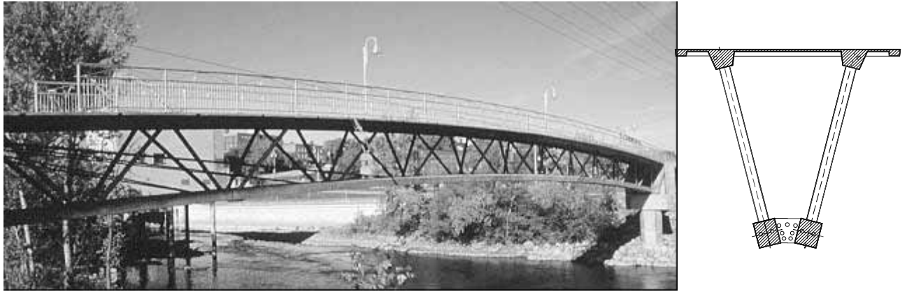
Figure 8 Sherbrooke footbridge, Canada,1997
