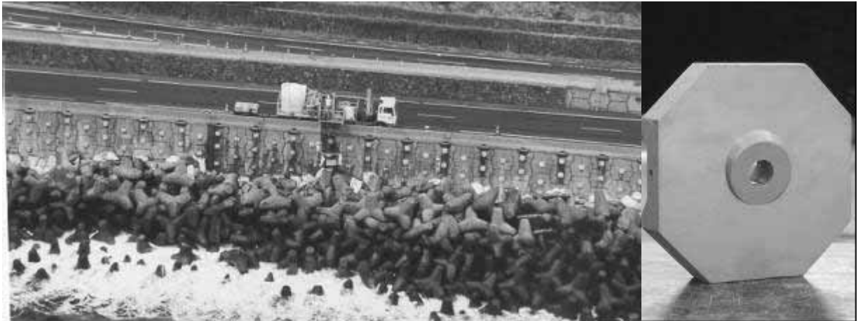
Figure 13. Ductal® retained earth anchors – La Réunion Island (1999)
