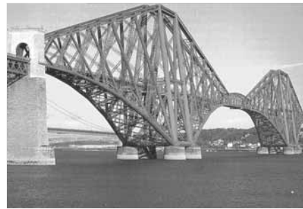
Fig. 5 The Forth Bridge
