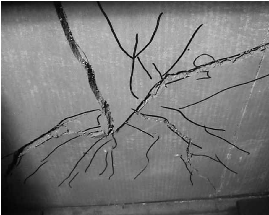
Figure 13: crack pattern in plate 5 (100 * 100 * 8 cm) centre load
