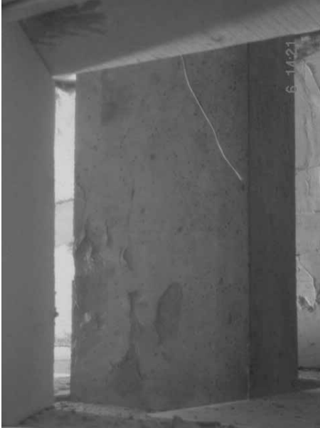
Figure 7: Spalling of concrete during the fire test
