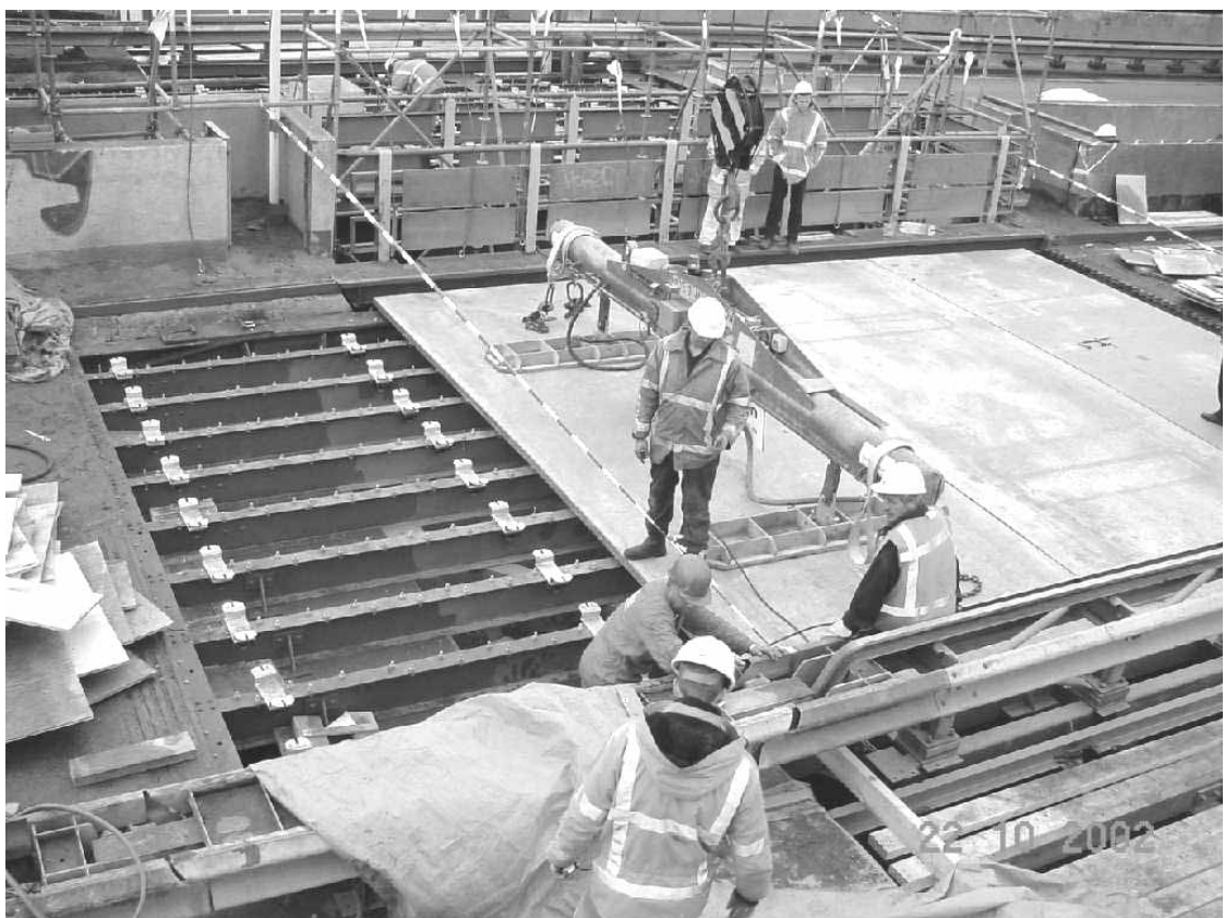
Figure 5: laying down the panels with a vacuum lifting boom
