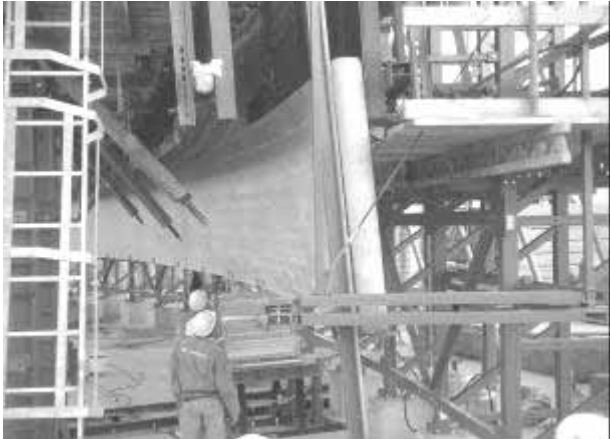
Figure 5: CERACEM BFM-Millau element (source: Eiffage)
