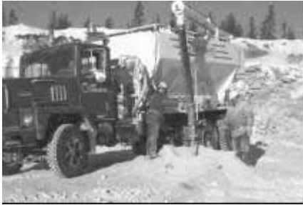
Figure 5 : Filling the blasthole
