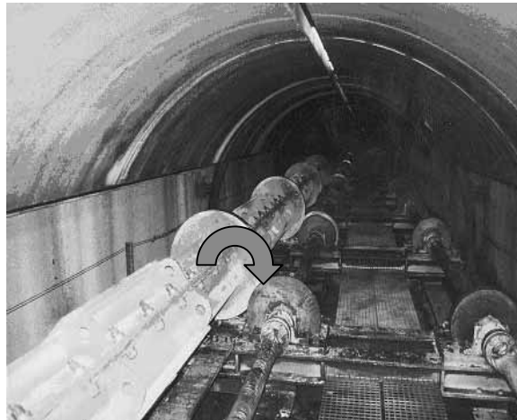
Fig.1 Centrifugation: production of a concrete pile
