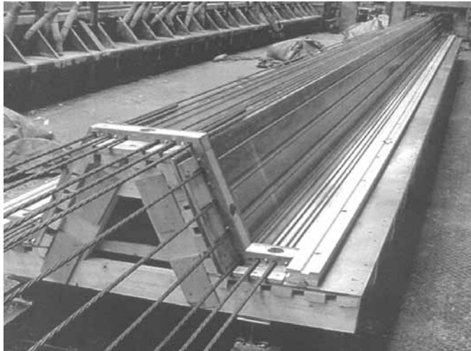
Fig. 7. Production of a prestressed sheet pile of UHSFC
