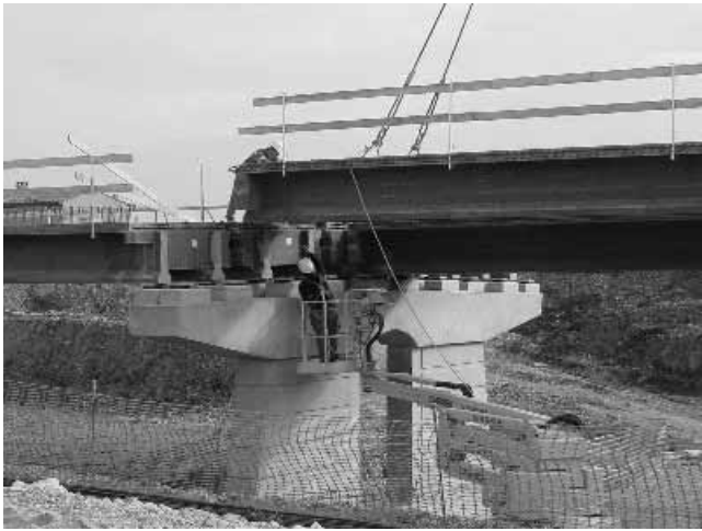
Figure 6: Erection of a precast beam
