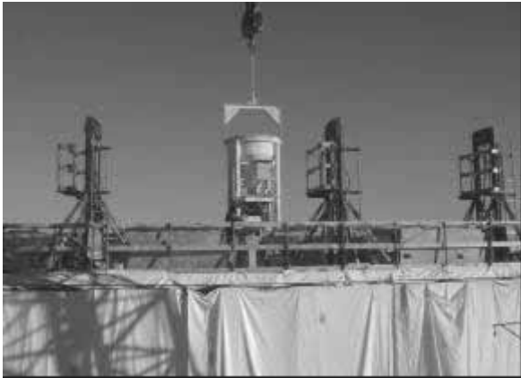
Figure 3: Element casting (source: Eiffage)
